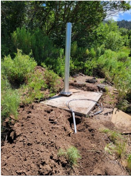
Concrete slab with solar mount pole
